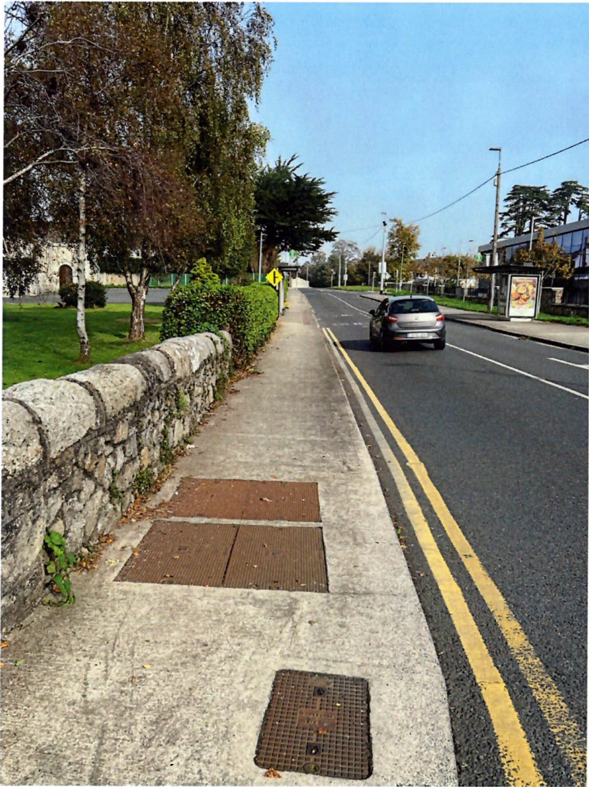
Figure 2 Shanganagh Road / Beechfield Manor Junction
